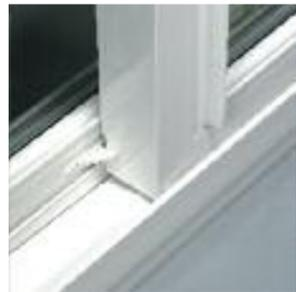
Sash vent stops allow fresh airflow.
